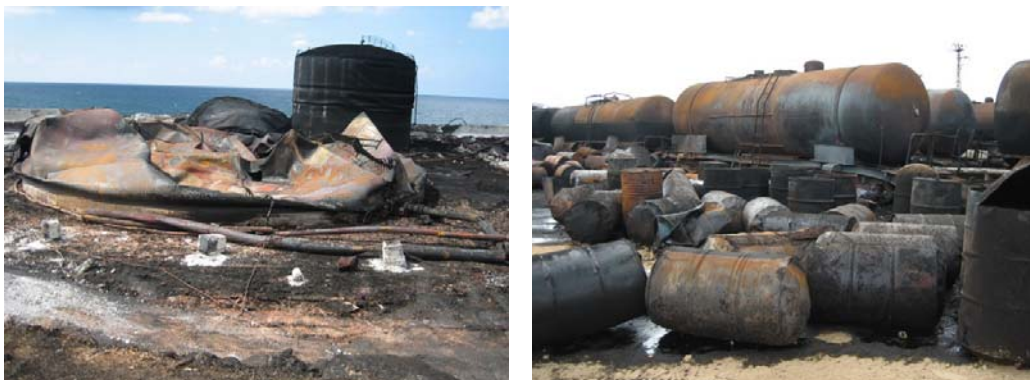
Figure 7.6. Different Types of Damaged Fuel Tanks in Jiyeh
